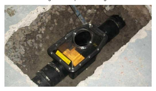
When you develop the basement keep the location of this access box cover in mind. If you should ever have a sewer backup, Aquatera Utilities and/or a plumber will want access to this device.
